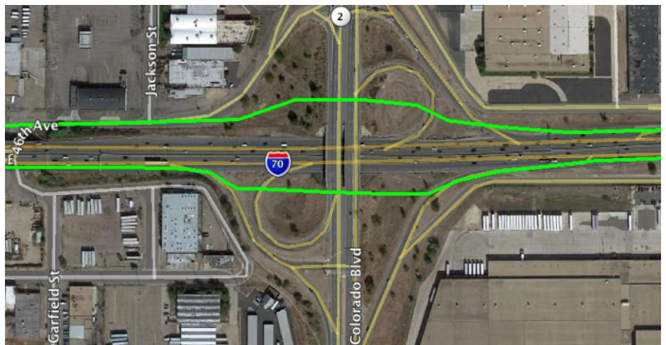
Colorado Blvd. Interchange
